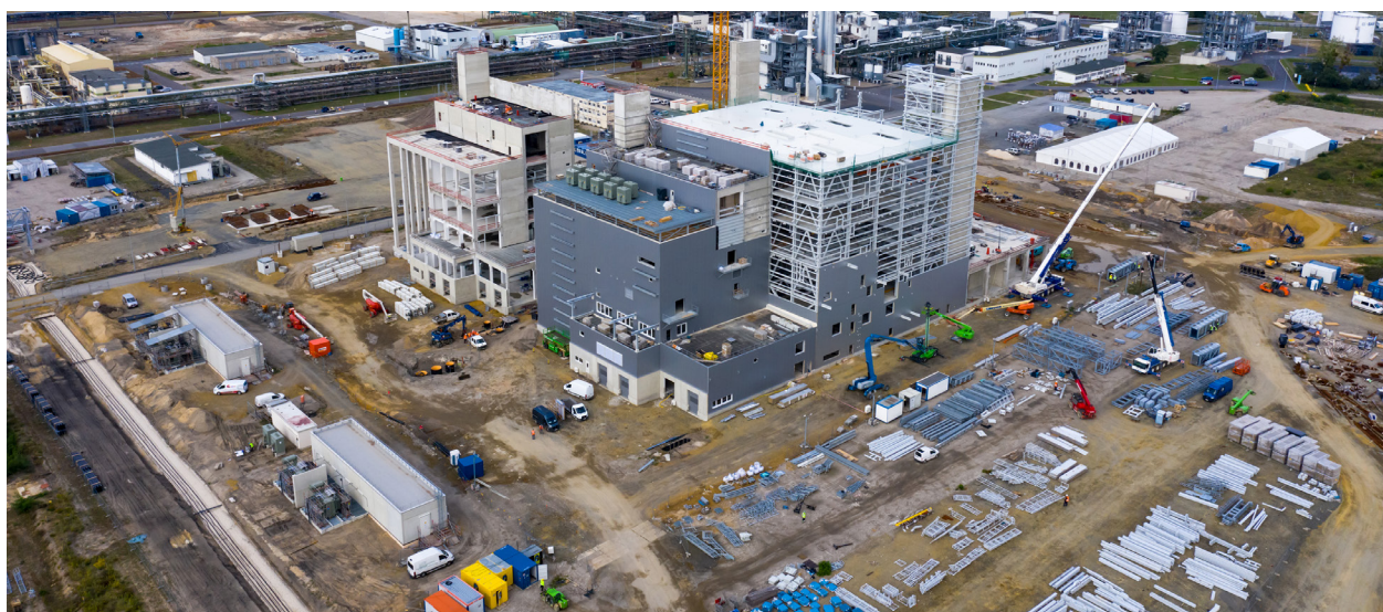
Figure 2: Construction of a stick-built plant (Source: BASF SE)
